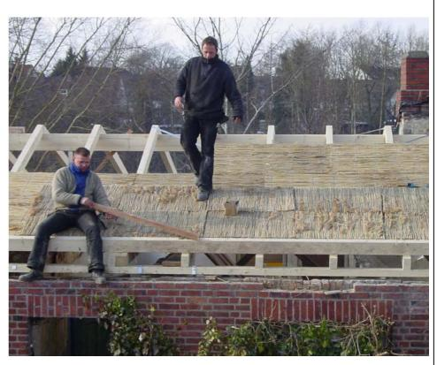
Reed upon the rafters used for roof insulation
