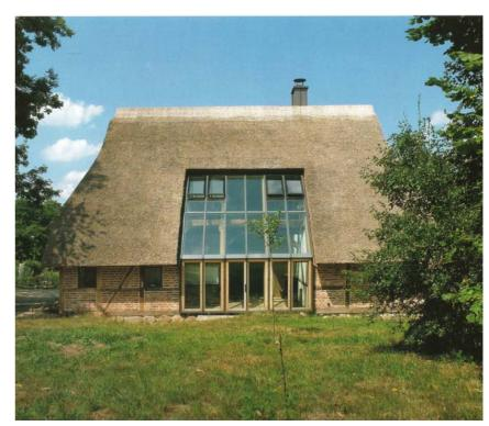
The south elevation of a north German reed roofed house. A conservatory delivers light and heat by the passive use of solar energy
